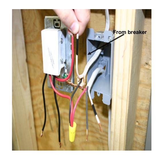
Attach the BLACK CYCLE wire from the thermostat (refer to step 1) to the BLACK wire from the heater.
