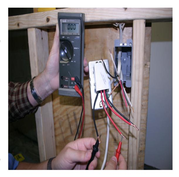
Attach the ground wire from the breaker and the ground wire from the heater cables to the green ground screw on the thermostat.
