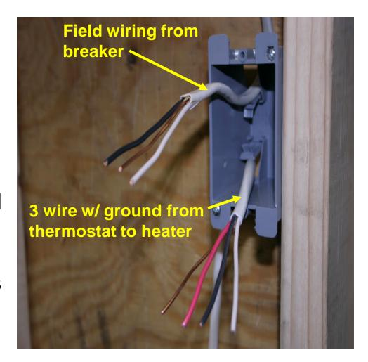
Notice the BLACK tape wrapped around the white wires from the breaker and the heater cables. This is to identify these wires as HOT wires instead of Neutral wires.
