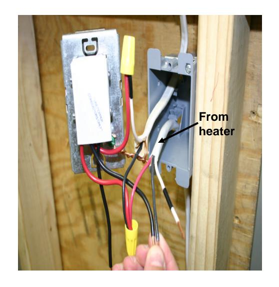
Attach the other BLACK wire from the thermostat to the WHITE wire (with black tape) from the heater.
