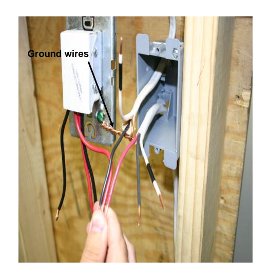
Tie together the BLACK wire from the breaker, the RED wire from the heater cable and the RED CYCLE wire (see step 1) from the thermostat with a wire nut.
